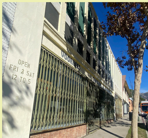
Washington Hardware Store (1403 N Lake Avenue) is constructed in 1930
