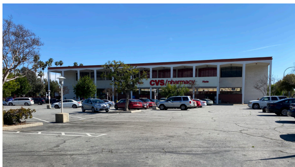
CVS and its surface parking which take up 3 acres in the northeast of the subarea
