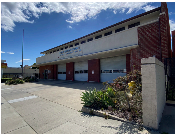
Fire Station 33, located in the subarea
