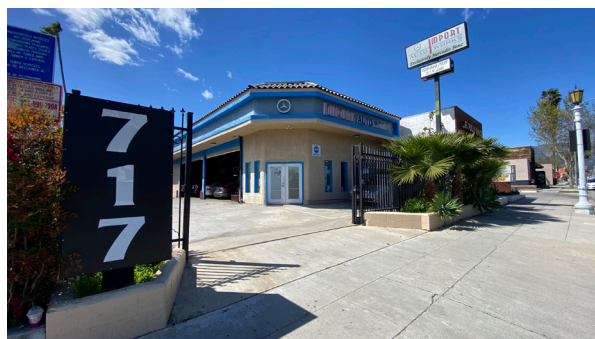
Vehicle repair business featuring a large driveway curb cut
