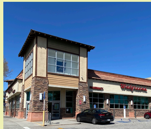
Walgreens Drug Store (670 N Lake Ave) is constructed in 2006
