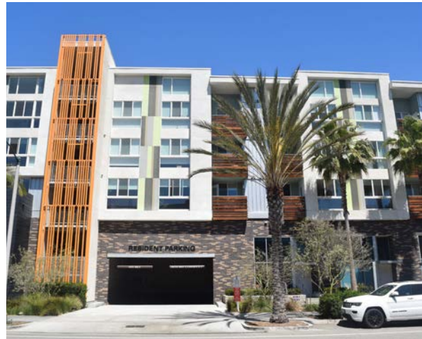
Housing options meet a variety of affordability and unit configuration needs for residents
