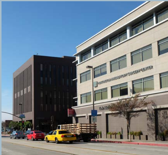
Medical office uses at Fair Oaks Ave and Congress St include 4-5 story buildings, several of which include non-transparent ground floors
