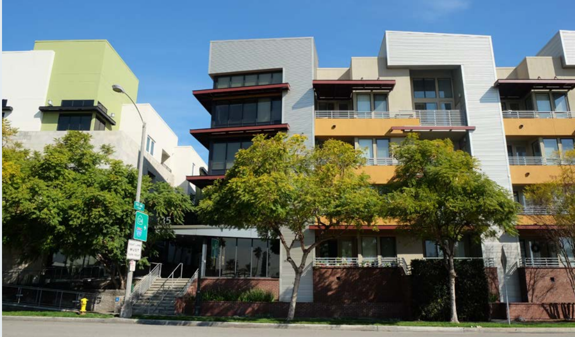
Balconies and other variations in wall plane depth create visual interest
