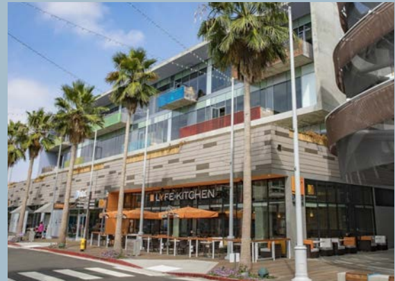
Integrated medical clinic in mixed use development with large second floor terrace that connects activity to the ground floor and creates an amenity for patients, employees, and visitors.
