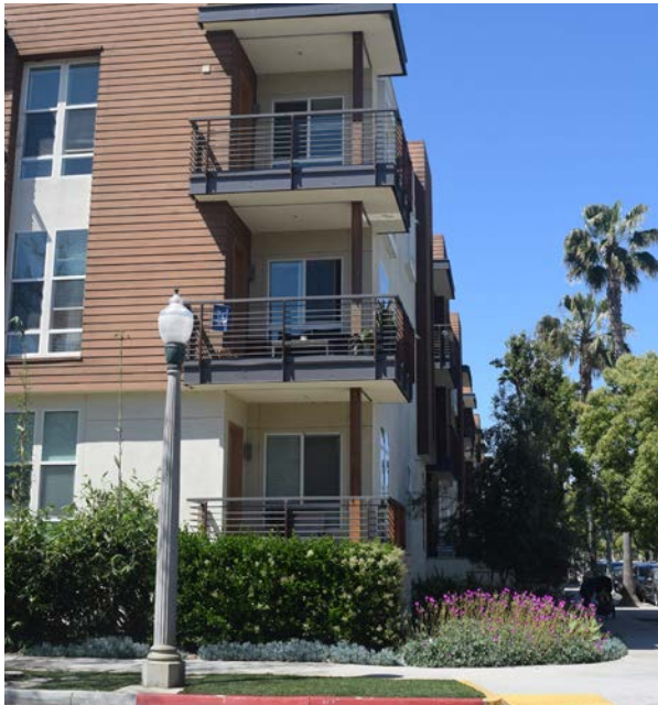
Private Open Space (Patio and Balconies)
