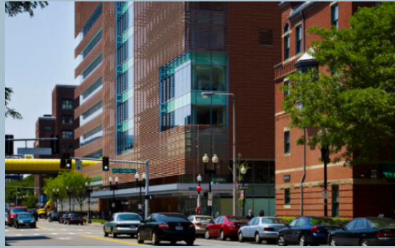
Medical office with exterior screen that reflects historic brick color and horizontal design
