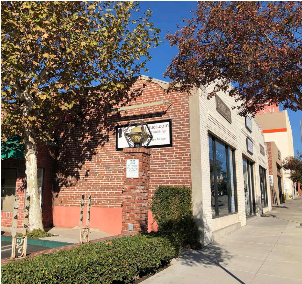
Adaptive re-use of pre-1940s buildings for commercial storefronts contributes to South Fair Oaks’ eclectic character
