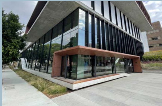
Ground floor landscaping surrounds a primary entrance and sets the building back from the street, protecting street trees
