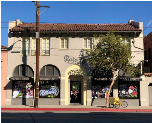
Simplified parking requirements allow greater flexibility for small businesses, especially in older buildings
