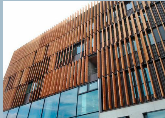
Medical research center with contemporary architectural features including wood screen and glazed facade
