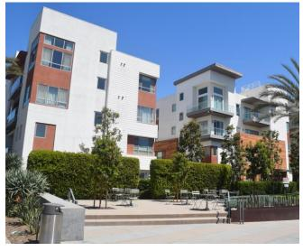
Façades over 50 feet in length and 2 stories in height shall modulate a minimum of 25% of the area above the ground floor at least 2 feet in depth.
