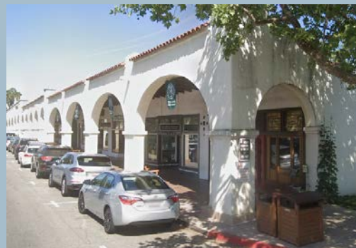
Galleries cover the sidewalk, but unlike arcades, the space above is not enclosed
