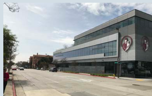
Healthcare Facility at 909 S Fair Oaks Ave (built 2017)
