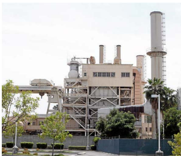
Power-generating facilities on the Glenarm Power Plant site
