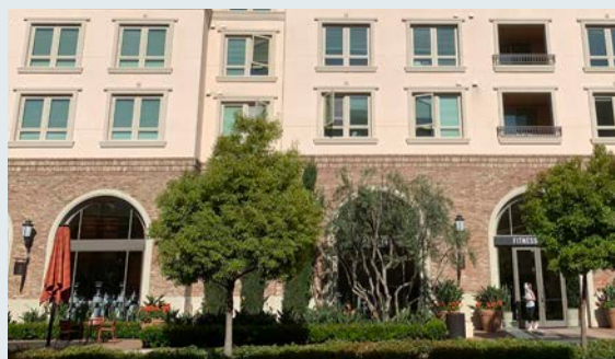
Ground floor frontage with combination of commercial and gym for occupants of residential building
