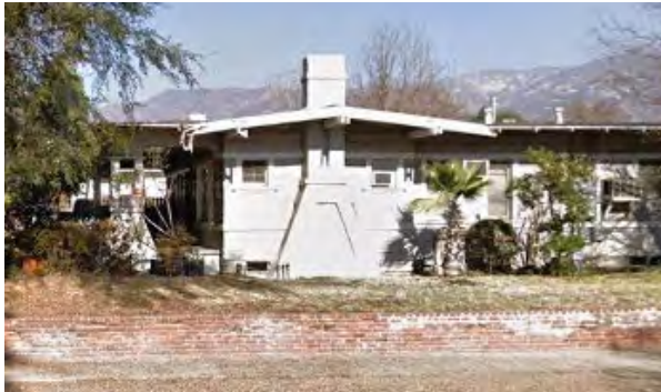
California Bungalow style house at 1826 Lincoln Ave.
