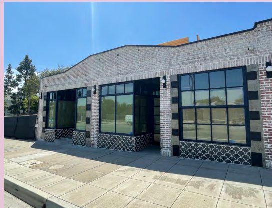
Commercial building on Lincoln Avenue using traditional materials and facade patterns.
