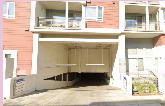
Example of parking entrance design without screening or façade integration.
