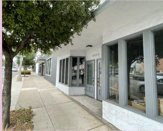
Commercial building on Lincoln Avenue with recessed entrance and transparency
