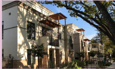
Balconies and other variations in wall plane depth create visual interest
