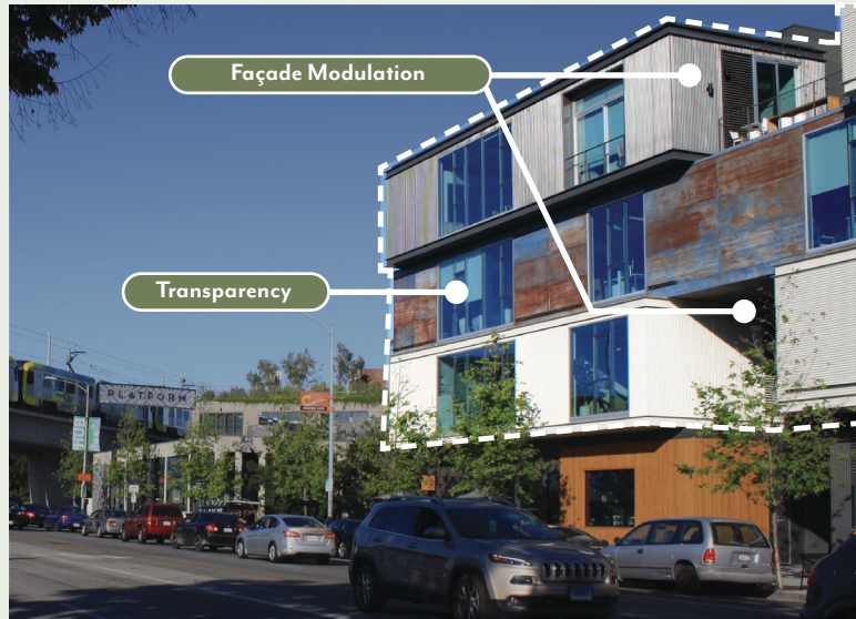
Façade modulation and transparency increase visual interest for R&D office buildings
