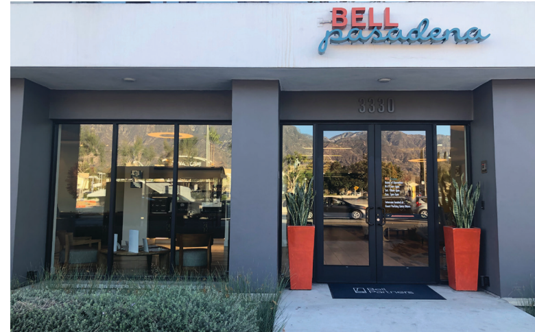
Example of appropriate ground floor transparency for a residential common area
