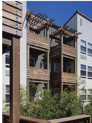
Private Open Space (Balconies)
