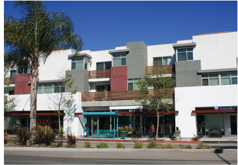
Example of approximately 39' foot building
