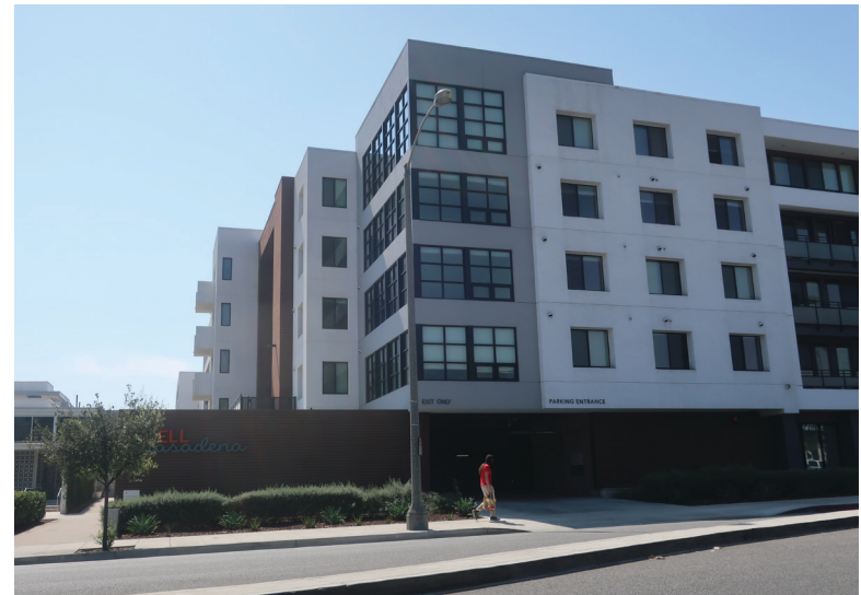
Example of approximately 56' foot building
