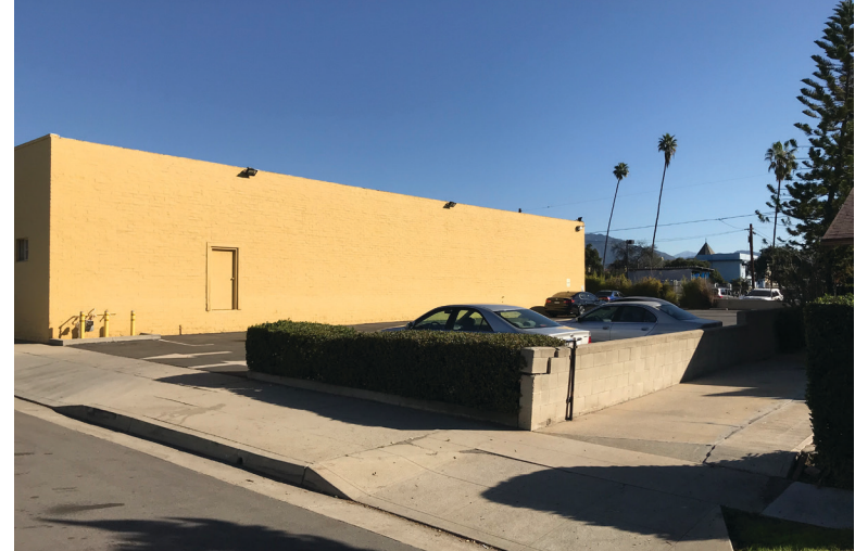
Example of a blank and windowless ground floor wall (Prohibited)
