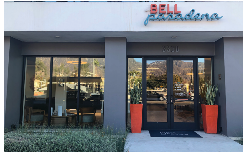
Example of appropriate ground floor transparency for a residential common area
