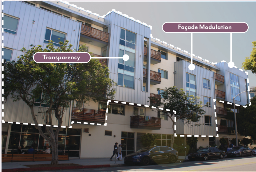
Variations in wall plane depth create visual interest and break up building massing
