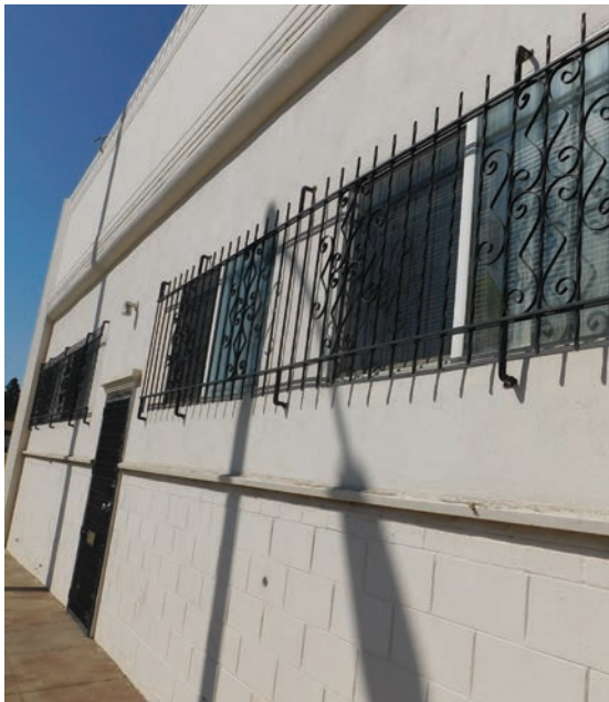
Example of exterior security bars (Prohibited)
