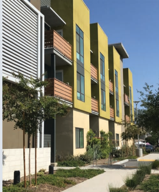
Example of approximately 39' building
