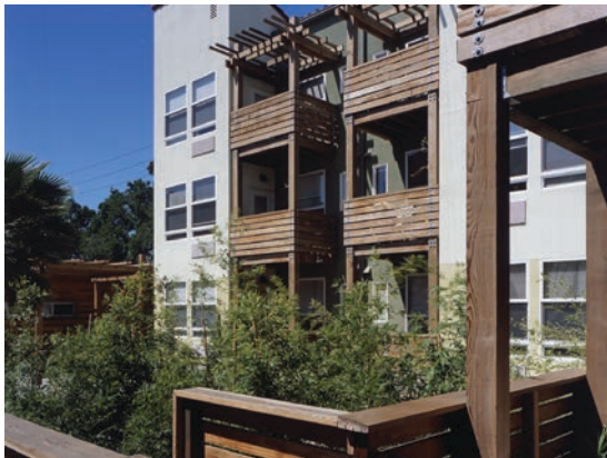
Private Open Space (Balconies)
