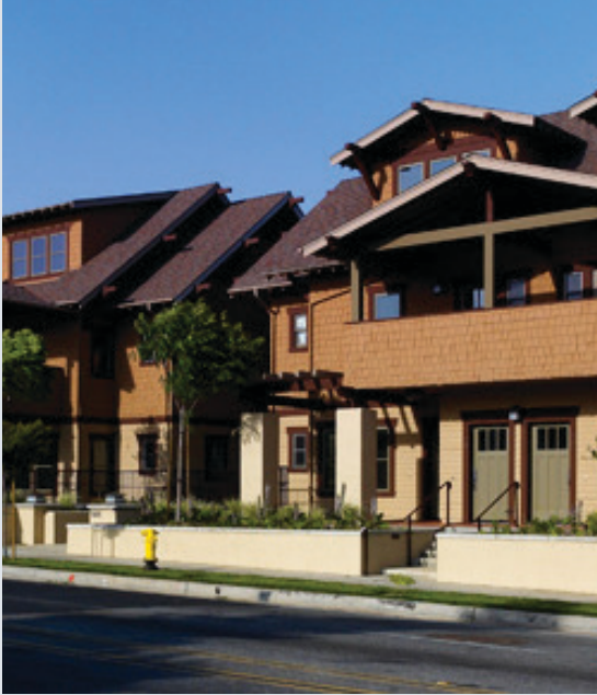
Example of approximately 36' building
