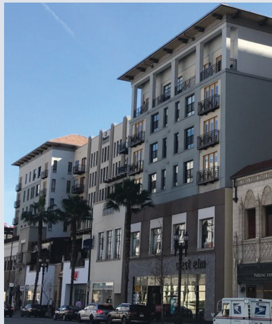
Example of approximately 75' building
