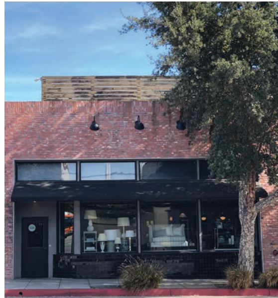
Example of appropriate ground floor transparency with a recessed entrance.
