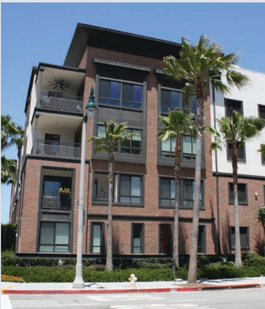
Example of approximately 51' building
