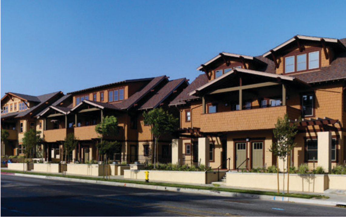
Example of approximately 36' building
