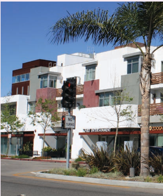
Example of approximately 39' building
