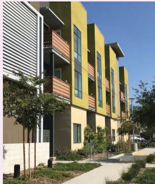
Example of approximately 39' building
