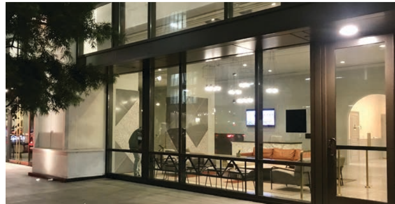
Example of appropriate ground floor transparency for a residential lobby (following non-residential requirements per section 6.4.3)
