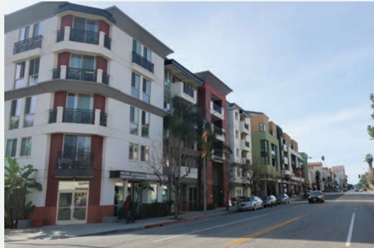
Example of approximately 55 foot building
