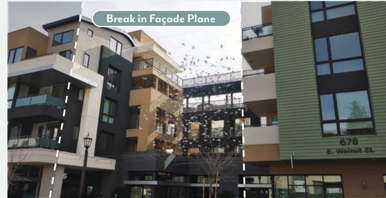
Suspended art can interact with a façade break to enhance the building entrance
