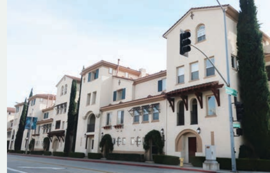
Example of approximately 45 foot building
