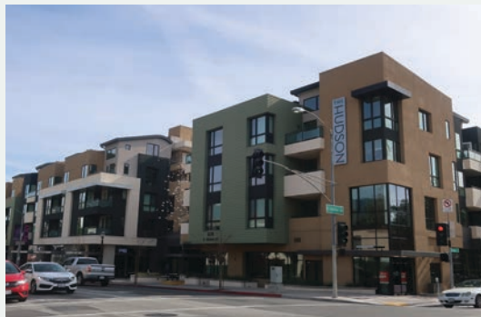
Example of approximately 50 foot building
