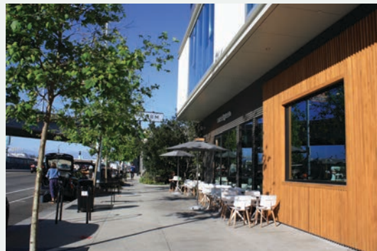
Example of Recessed Ground Floor
