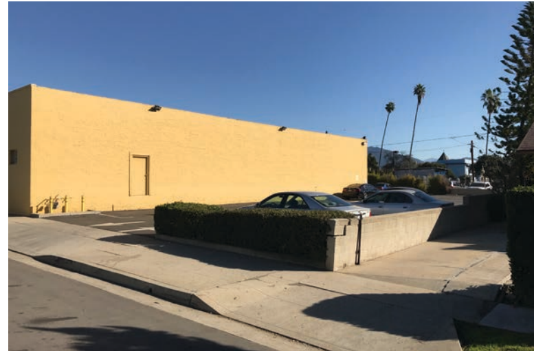
Example of a blank and windowless ground floor wall (Prohibited)
