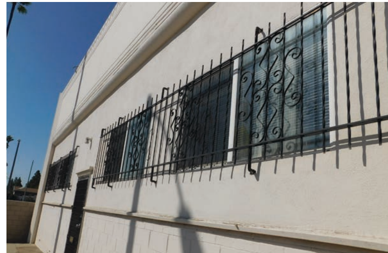
Example of exterior security bars (Prohibited)
