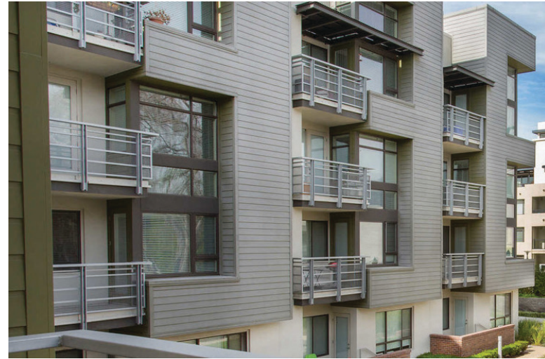
Private Open Space (Balconies)
