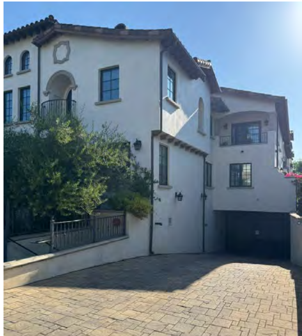
Materials do not change at this parking entrance; the same architectural style should be employed throughout
