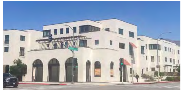
A new mixed-use development at Orange Grove Boulevard and Lincoln Avenue
