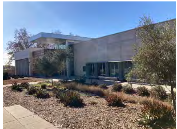
The Robinson Recreation Center provides an open space and a variety of community programming
