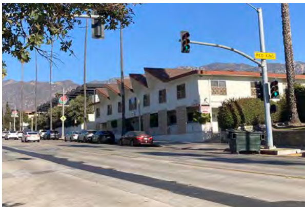
Signalized pedestrian crossing are located at major intersections
