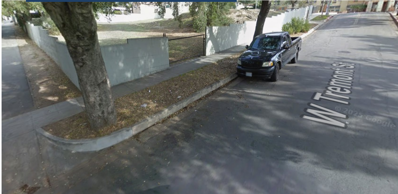
Sloped condition on Tremont St (west of Fair Oaks)
