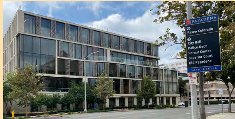
Emphasizing the horizontal dimension can make a tall building appear less overwhelming.
