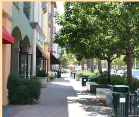
Wider walk zones of at least 7 feet are appropriate for commercial retail areas.
