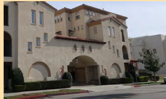
Entrances integrated in the architecture of the building reduce the visual impacts of parking.
