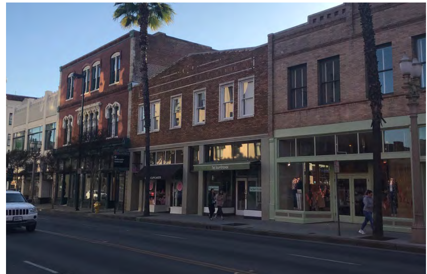
Traditional storefronts and historic architectural styles on North Fair Oaks Avenue
