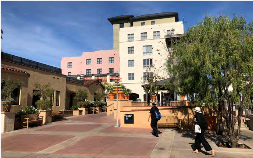
Public plaza and transit-oriented development at the Del Mar Metro station
