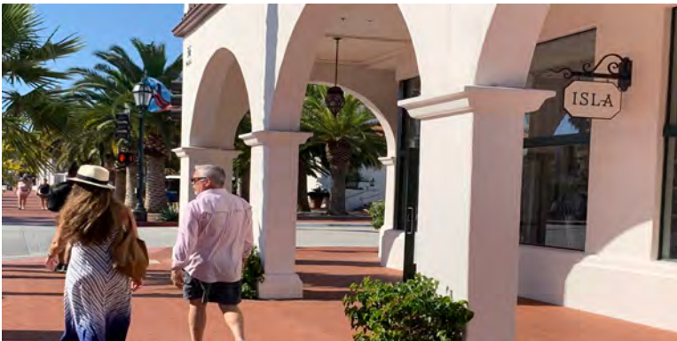
Arcades can provide additional cover for pedestrians.
