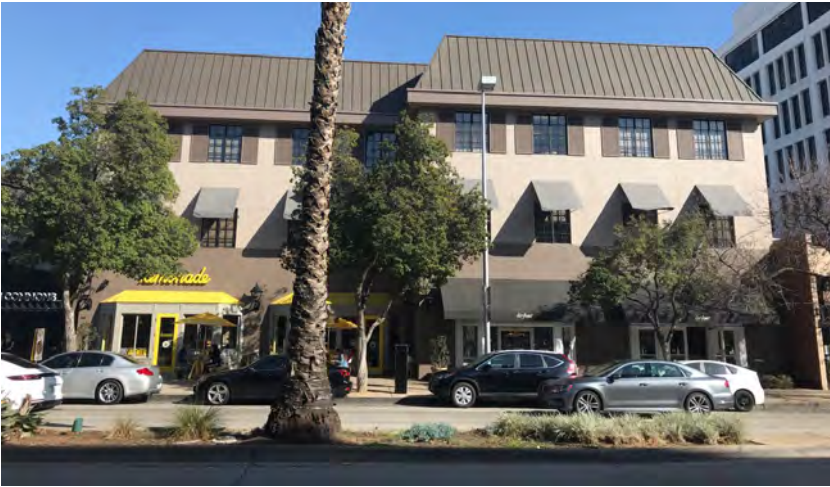
Mixed-use building with retail storefronts along Lake Avenue and landscaped median in the foreground
