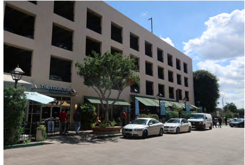
Parking garage with ground floor retail, street furniture, and landscaping along Shoppers Lane
