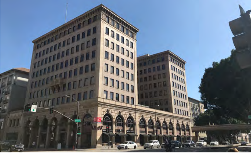
Historic office building in Civic Center Financial Historic District
