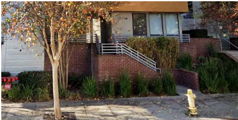
Side of a stoop set back from the sidewalk line by a planted area.
