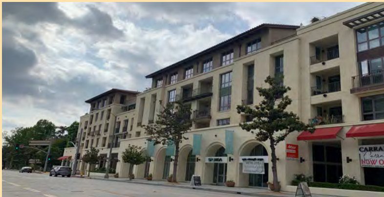
Three dimensional character should vary as a building rises skyward; differentiate between the base, middle and top levels of a building.
