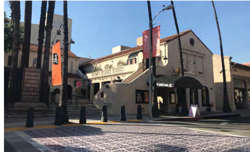
Historic Pasadena Playhouse and Engemann Family courtyard on El Molino Avenue with decorative crosswalk in foreground
