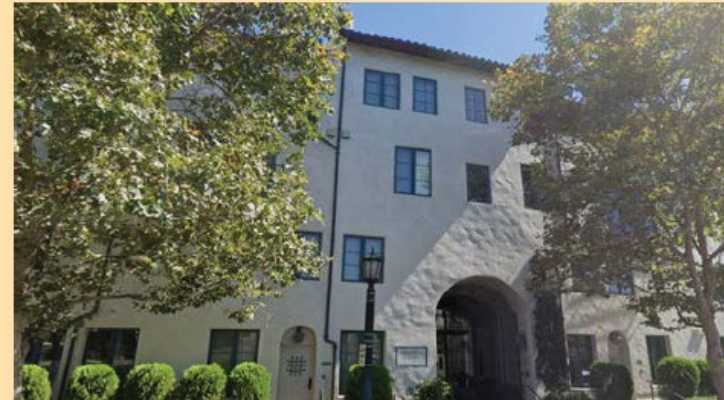
Well-designed downspouts using high-quality materials.
