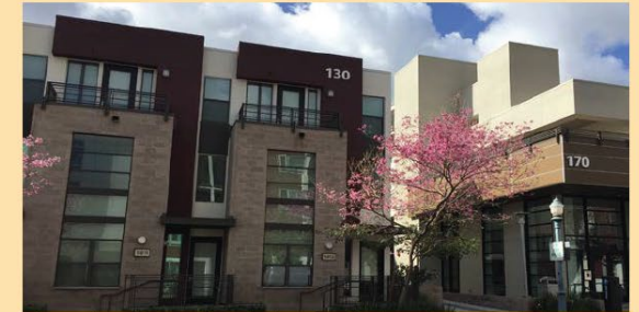
The number of materials and colors should be limited; where multiple materials or colors are used on a façade, they should transition at inside corners.
