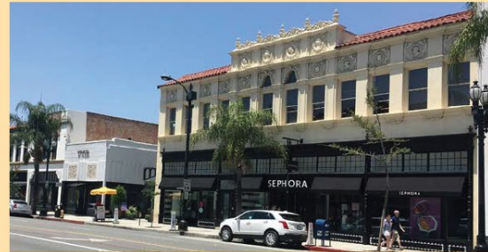
A hierarchy of vertical and horizontal expression should be used; façade articulation should reflect changes in building form.
