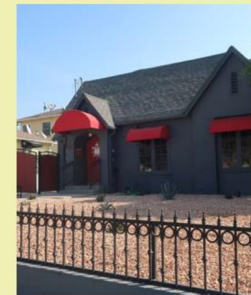
Adaptive re-use of Spanish Colonial Revival/Spanish Eclectic residential building to commercial office
