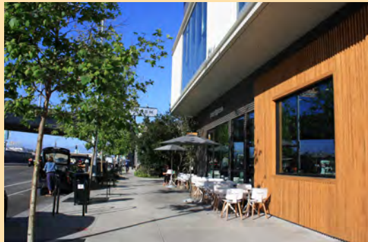
A recessed ground floor can provide additional shade for pedestrians or building users while allowing space for other amenities
