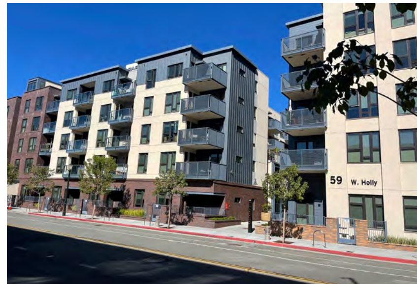
5-story mixed-use development along Holly Street west of Fair Oaks Avenue
