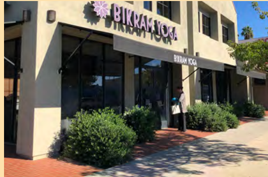
A three-to-five foot setback allows for more significant landscaping at the sidewalk
