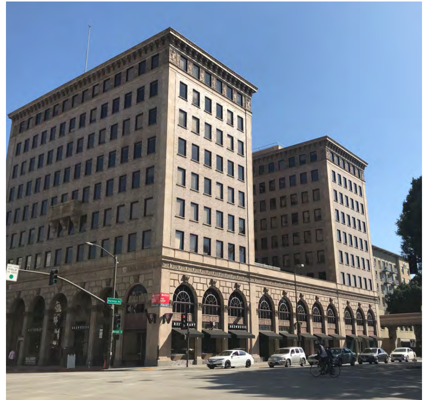
Pacific Southwest Building at Colorado Boulevard and Marengo Avenue, in the Civic Center Financial Historic District
