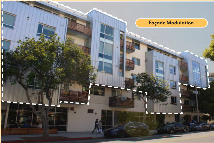
Balconies and other variations in wall plane depth create visual interest
