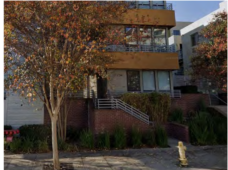
The side of a stoop set back from the sidewalk line by a planted area
