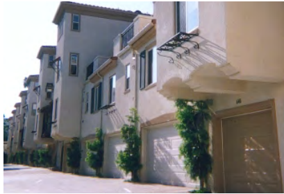
Downtown Precedent: parking garages front on a drive rather than the street
