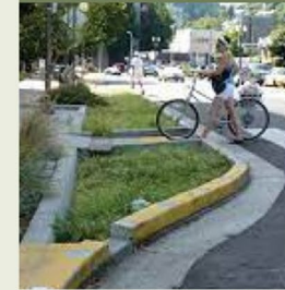
Curb extensions (or bulb-outs) increase sidewalk width and can contribute to traffic calming
