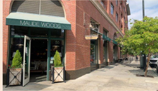
Ground floor frontage with commercial use, shade awnings, and a transparent entrance
